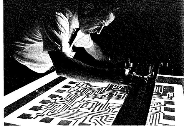
Fig. 4—Ruby being cut for custom integrated circuit designed by EASD engineers.
