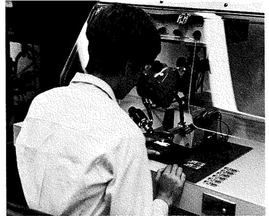
Fig. 7—Solder reflow process equipment for attaching cased devices to substrate.
