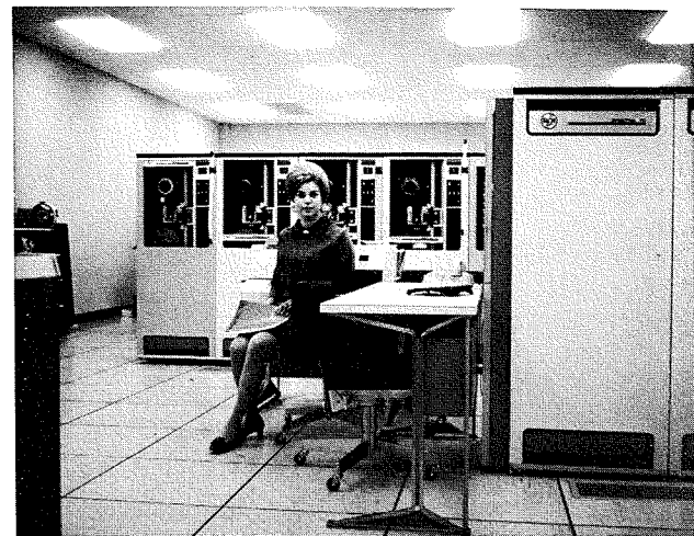
Properly planned computer site is well lighted, has underfloor air supply system, and is spacious.
