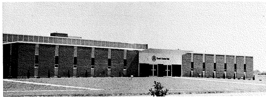
South Central Bell's Shreveport accounting center—a facility built around computer site.
