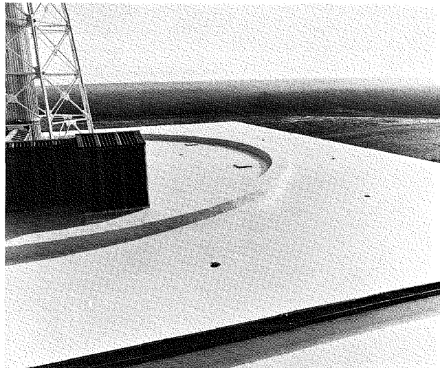
View of completed roof.
