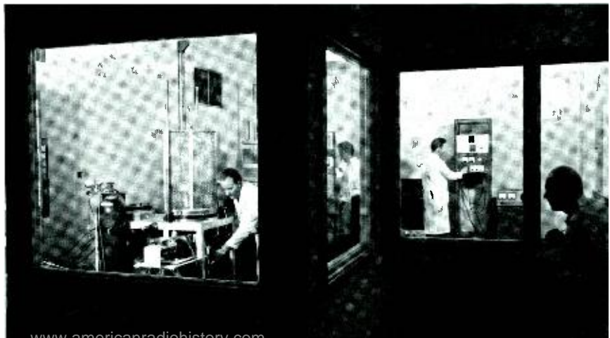
Fig. 10—White room and facilities for superconductive thin film fabrication.
