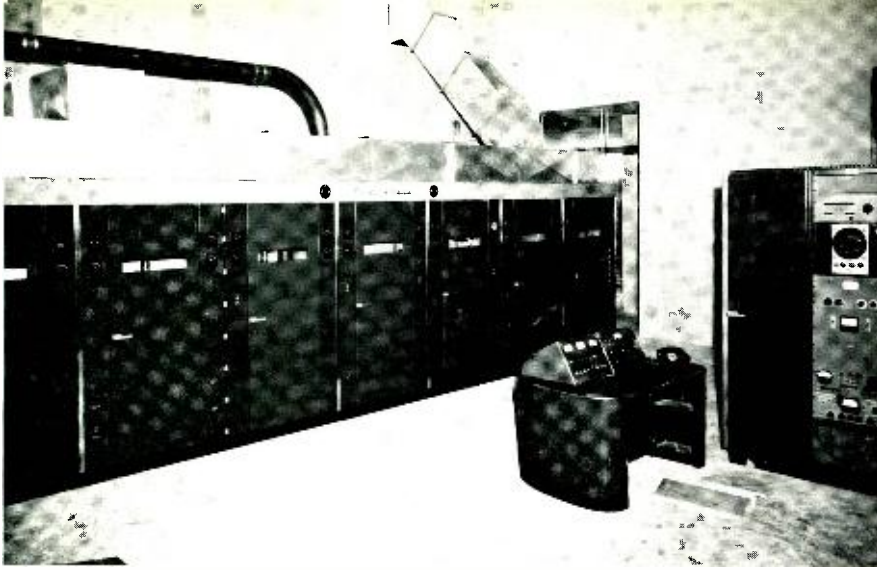
Fig. 3—Front line of 7 aluminum cabinets containing the r-f circuits.
