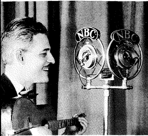
Fig. 1—Kelvin Keech performing before a pair of Western Electric carbon-button microphones. Because of unpredictable "packing," these microphones were used in pairs to improve reliability. (Early 1920's).
