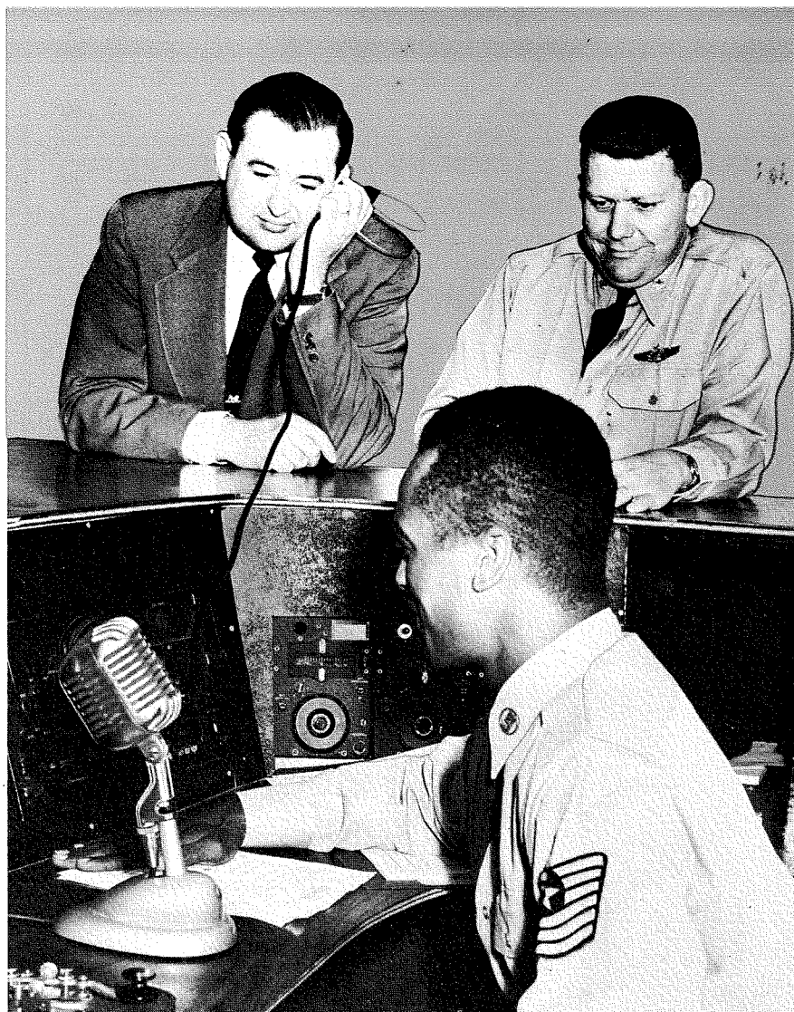
Fig. 3.—RCA Field Engineer Al Pontus listens while control tower operator checks installation of communication console equipment.
