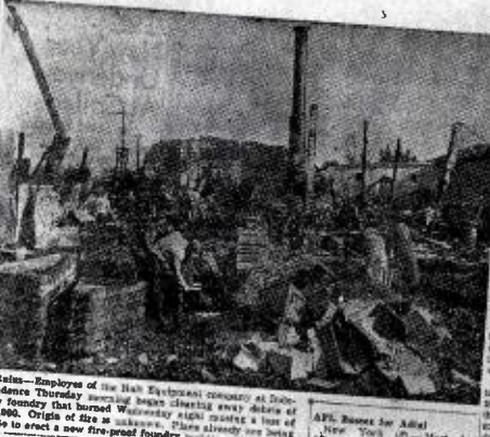
Rains—Employees of the High Experimental Company at Independence Thursday evening were clearing away debris of new foundry that burned Wednesday night causing a loss of $75,000. Origin of fire is unknown. Plans already are being made to erect a new fire-proof foundry.
