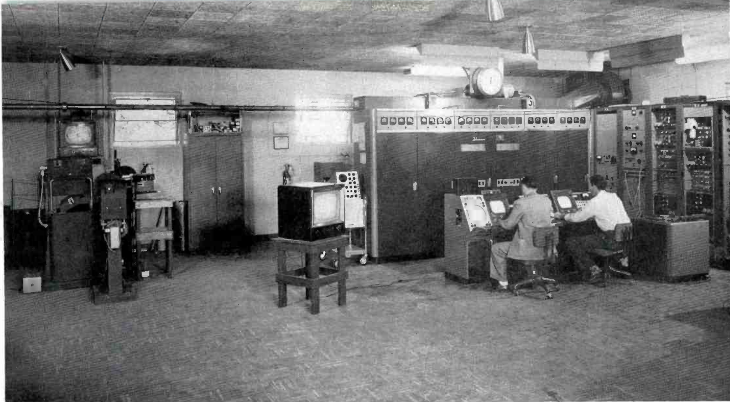
TRANSMITTER ROOM. shown above, houses RCA TTU-1A Transmitter (right center) and control racks (far right). This room was purposely made large enough to allow for addition of 10-kw amplifier at a later date. At the present time, the station film equipment (far left, above) and film and network control equipment (combined with transmitter desk) are also located in this room. With an enclosed announce booth (not shown) this provides for complete operation from this point until KPTV's studios are completed.
