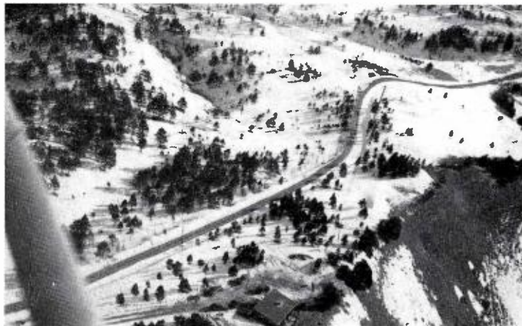
FIG. 10. Aerial view of the KOZY Transmitter House (bottom of photo), and the "Skyline Drive" approach.
