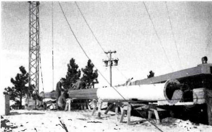
FIG. 9. View of the Pylon FM Antenna during assembly prior to installation.
