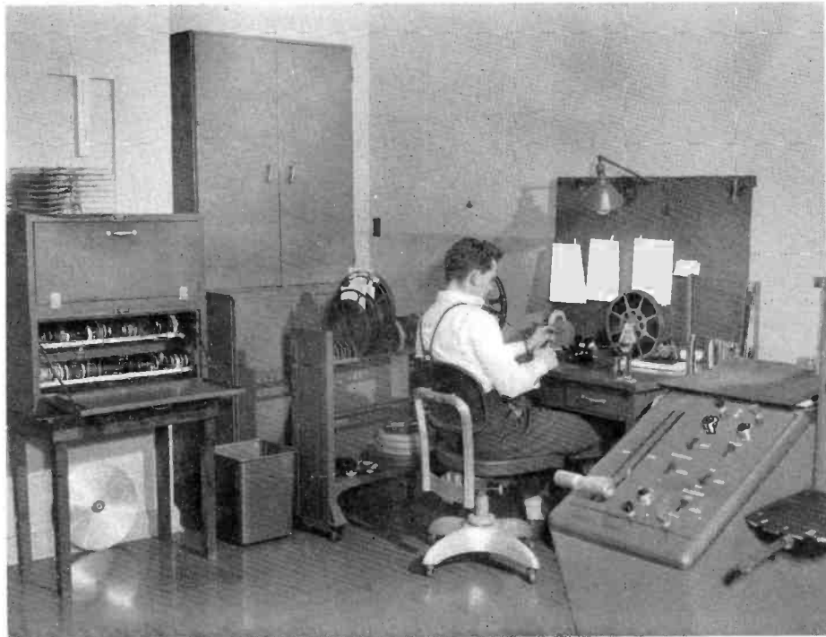
FIG. 7. WDAF-TV film projection room showing two 16mm projectors and the Gray Telop for transmitting the opaque slides. An RCA receiver is used as a line monitor. Note covered floor-trenches which carry all wiring for the projection equipment. These trenches were installed in many parts of the building, even to outside walls for future expansion.
