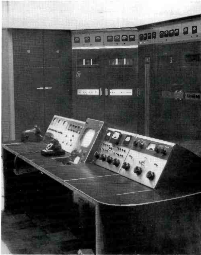
FIG. 10 (above). The 10 KW RCA FM Transmitter and the 5 KW RCA TV Transmitter are arranged in line with the left and right ends, respectively, bent around so that the equipment units form a shallow U. In the center of the U is the combined control desk. The view above shows the control desk and left side of the FM transmitter.
