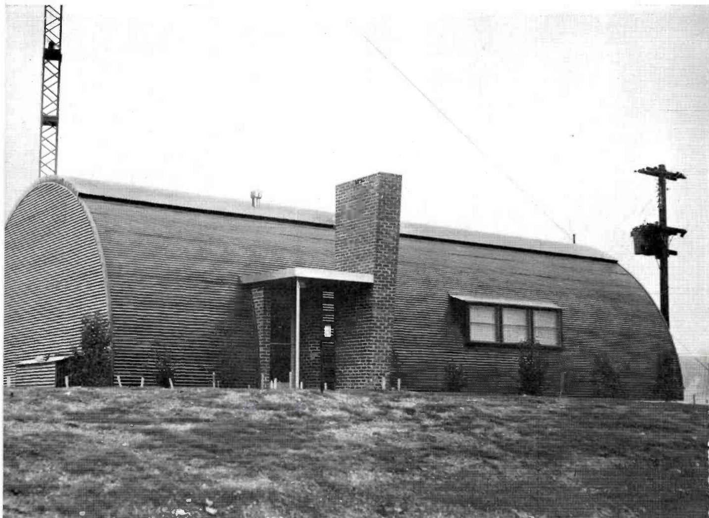
FIG. 9. The transmitter building is a modified Quonset, painted dark green and provided with brick trim which gives it a modern and pleasing appearance. In addition to the transmitter room it houses office, work shop, kitchen, storage space and rest room.
