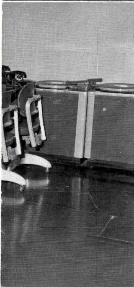
FIG. 5. View of the audio and video console in master control. Camera switching as well as master switching is performed at this console. Operators work entirely "blind." The RCA receiver is an "off-air" monitor.
