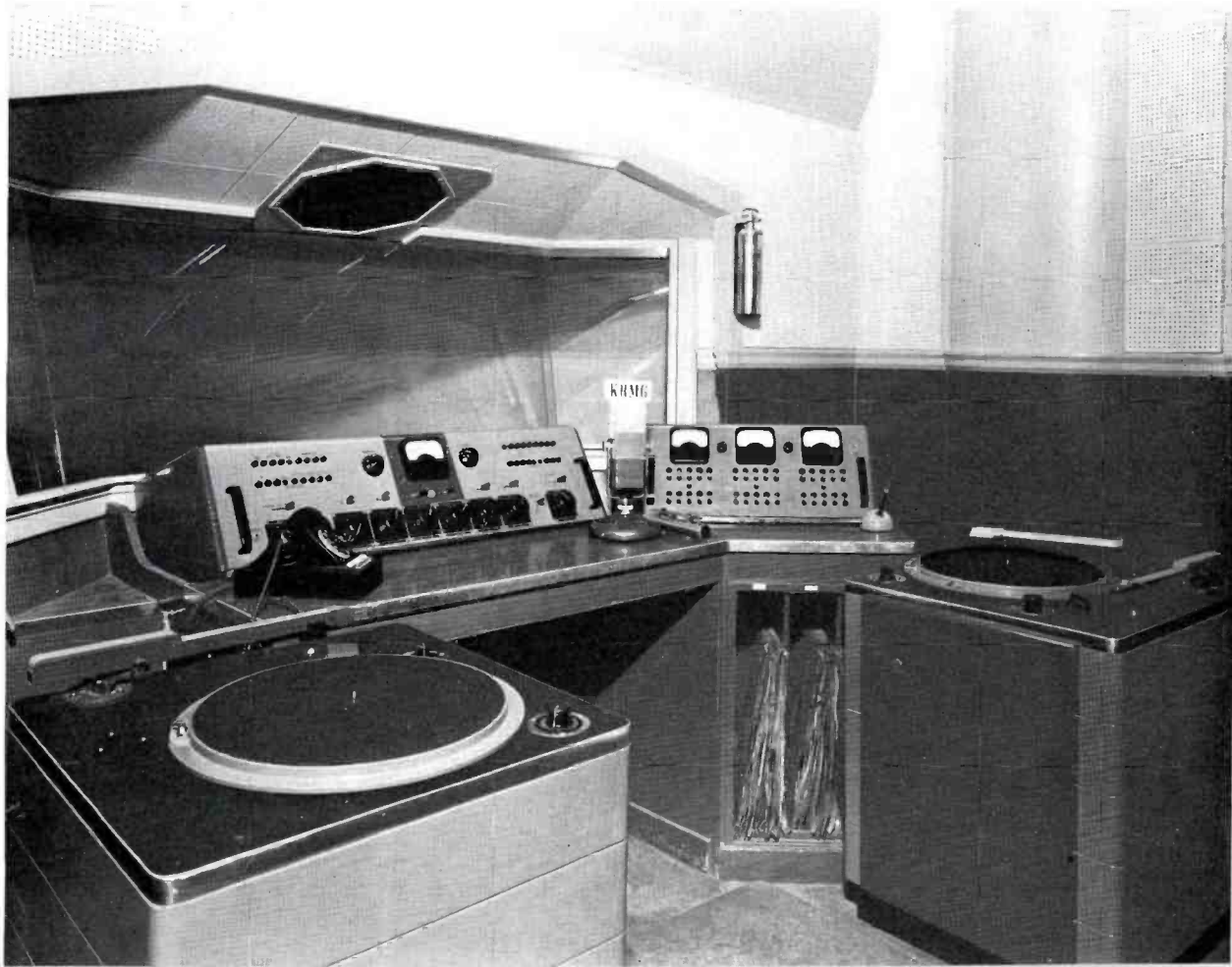
FIG. 5. View of Master Control Room of KRMG, looking into studio B. A Type BCS-1A Master Switching System is located to the right of the 76-C Console. Note location of LC-1A Speaker above the control room window.
