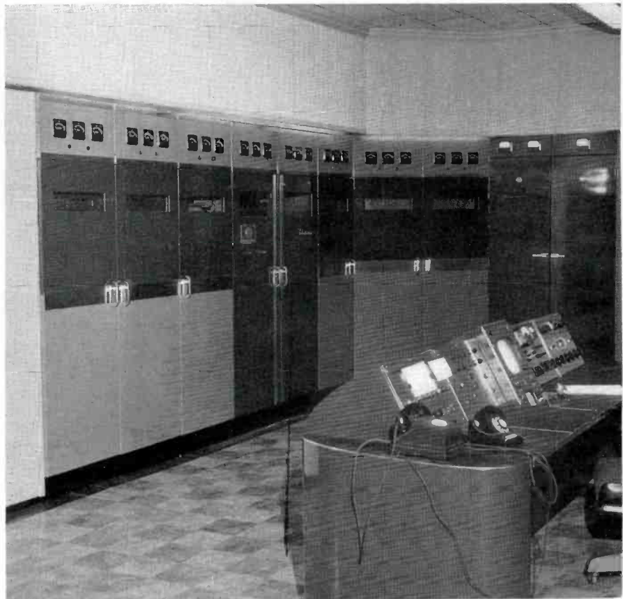
FIG. 10 (above). The 10 KW RCA FM Transmitter and the 5 KW RCA TV Transmitter are arranged in line with the left and right ends, respectively, bent around so that the equipment units form a shallow U. In the center of the U is the combined control desk. The view above shows the control desk and left side of the FM transmitter.
