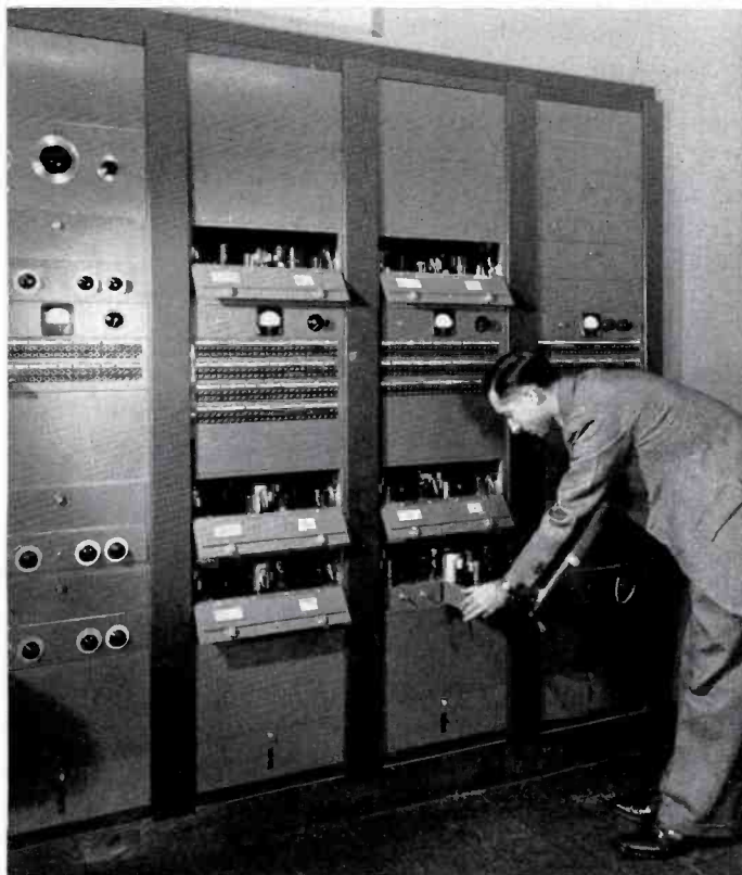
FIG. 3. Closeup of a section of the Master Control audio racks showing how all amplifiers, individual controls and components are easily reached. Plug-in type amplifiers are used throughout.
