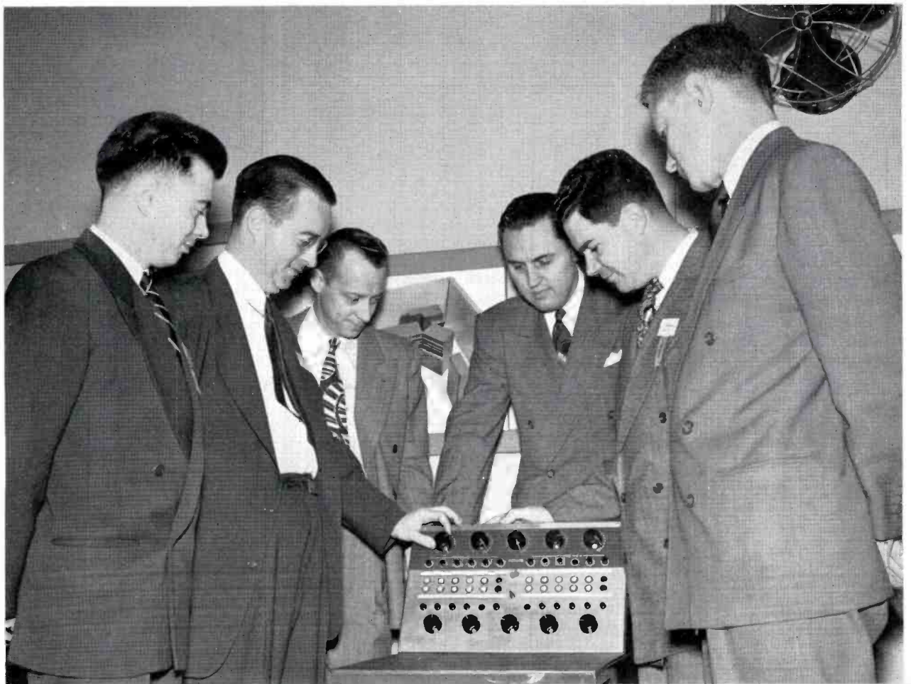
FIG. 2 (above). Norman Bean (back to photographer) gave members of the television clinic very practical pointers on operation of the Image Orthicon TV camera and camera control equipment. Broadcasters were then given an opportunity to operate the various units under his guidance.
