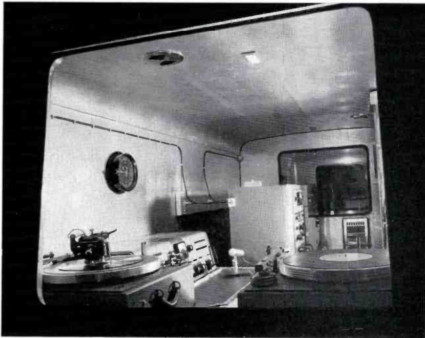
FIG. 2. This view through rear window of the mobile unit shows the location of the transcription recorders, the 76B-5 Console, and the transmitter and the monitoring racks.
