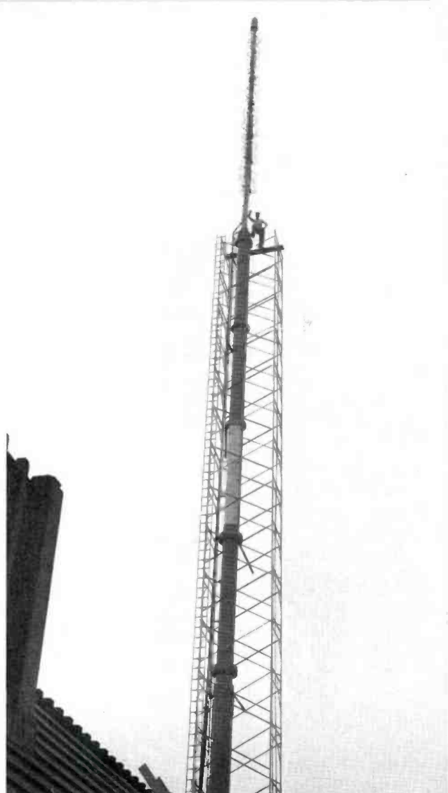
FIG. 25 (above). The Pylon sections were brought up one at a time. As each one was brought up it was stacked on top. Finally the Superturnstile was brought up (in one piece) and placed on top.
