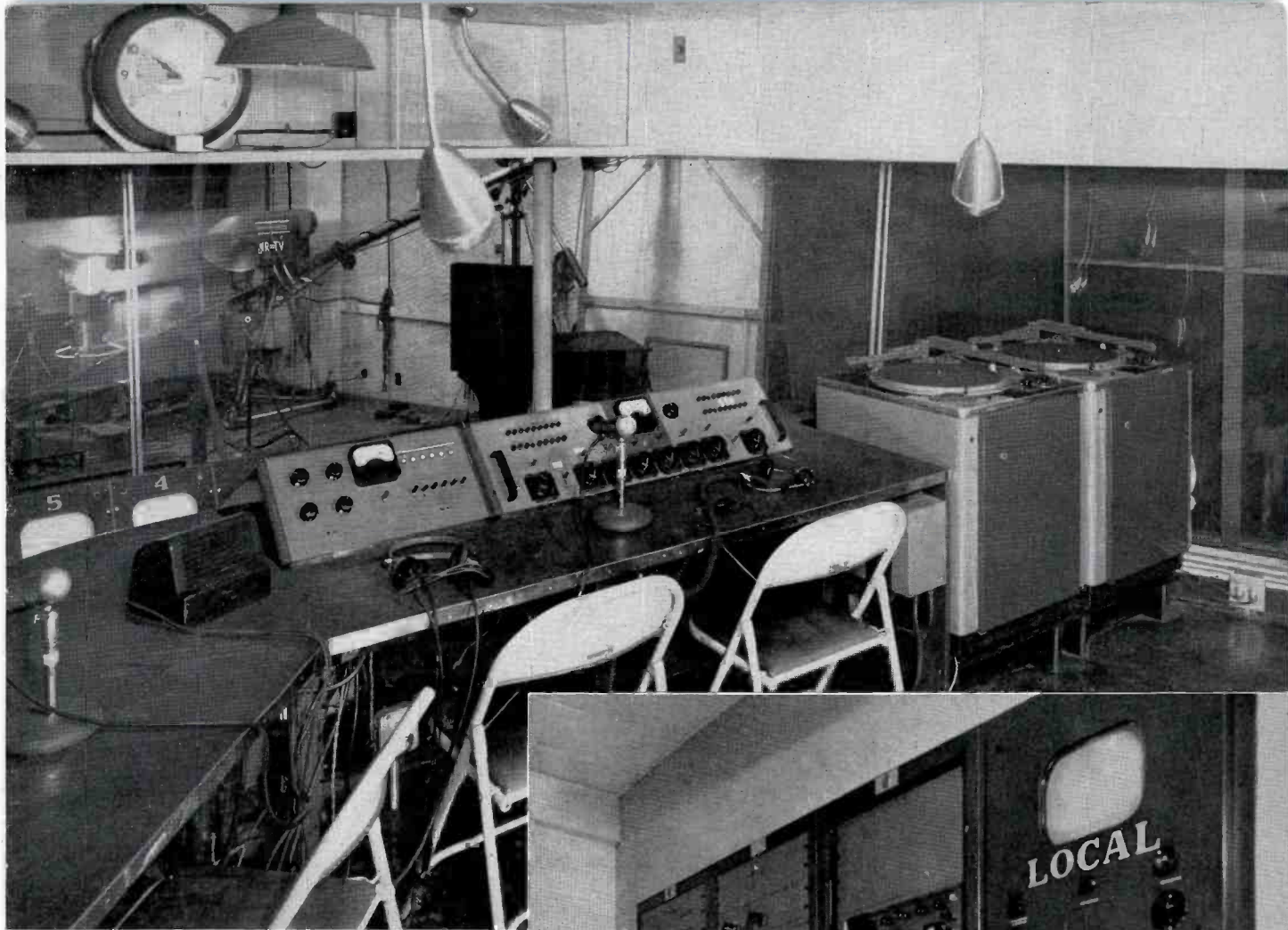
FIG. 11 (above). This view shows the arrangement on the upper platform to better advantage. Program director sits at the left, technical director in the center and audio operator at the right.
