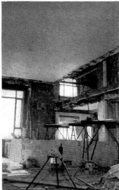
FIG. 6 (below). This is the control room corner of the penthouse studio during construction. Drop-ceiling type construction was employed in this two-story high studio.
