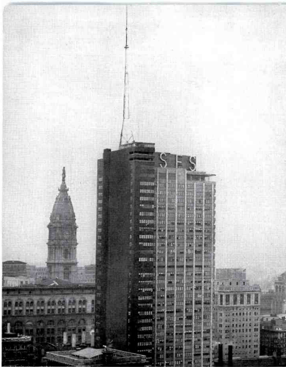
FIG. 23 (left). WCAU-TV's superturnstile antenna and WCAU-FM's two-section pylon antenna are mounted on top of a 181-ft. tower which surmounts the 479-ft. PSFS Building. Note famous statue of William Penn on City Hall in background.
