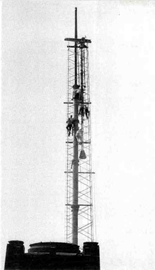
FIG. 24 (above). Erecting the antenna on the roof of the building was quite a problem. It was solved by building a tower-like scaffolding above a hole cut in the roof and bringing the sections up through the center of the scaffold.
