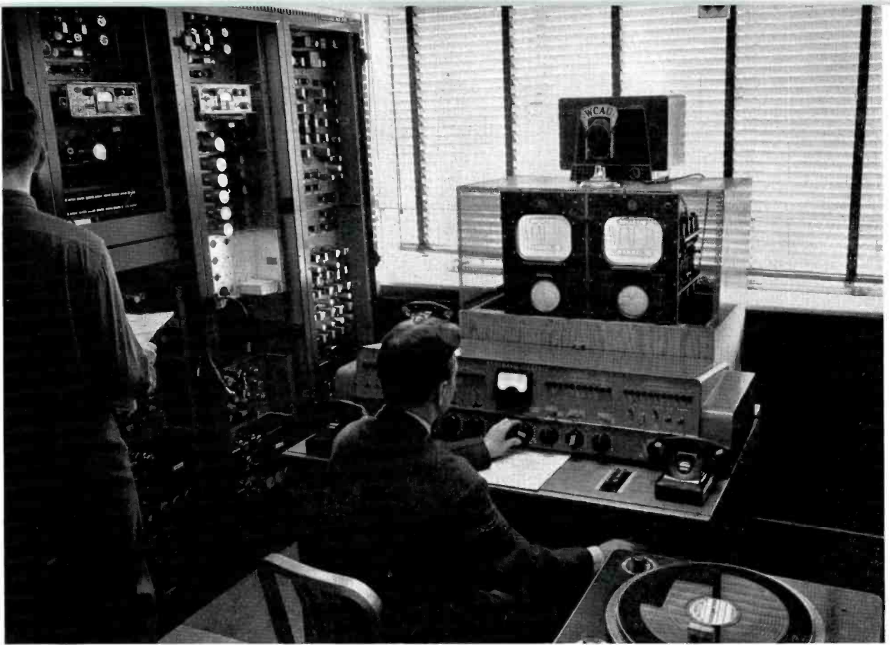
FIG. 28. View in the TV control room adjacent to the transmitter room. Operator sits at the desk containing video and audio monitoring and switching facilities. Terminal equipment and amplifiers occupy racks on either side.
