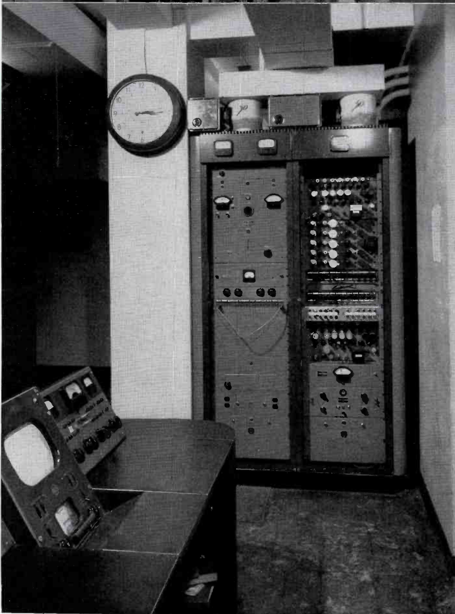
FIG. 19 (above). The view above shows the FM end of the transmitter control room (see floor plan, Fig. 8). The RCA BTF-10B FM Transmitter is at the right. At the left are racks containing audio and monitoring facilities, power supplies, etc. Turntable used for FM fill-ins and for testing is in the center. In the foreground is a corner of the TV transmitter control console.
