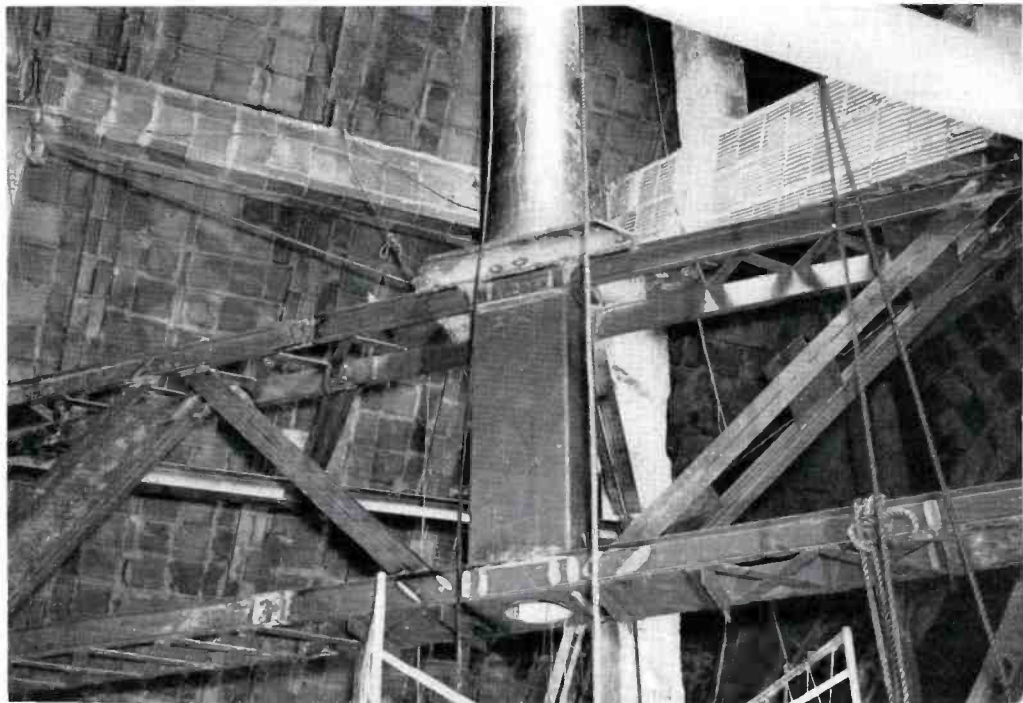
FIG. 26 (right). In order to secure the antenna supporting section onto the building the framework of the latter was reinforced and the welded steel frame shown here was mounted within.
