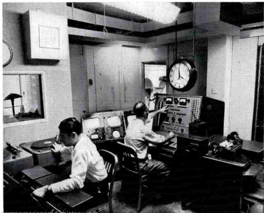
FIG. 15. Another view of master control room. Film camera controls are at left, turntables next, followed by video monitors (line, preview, on-air) and master switching console.
