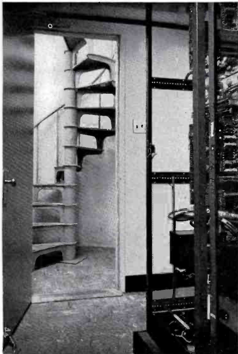
FIG. 13. The circular stairway which leads from master control to studios and control rooms.
