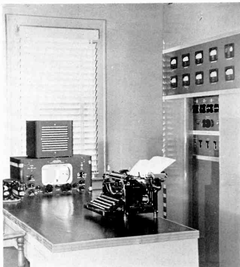
The RCA 250-K at WSAV. Speech input racks are located at the left of the window.
