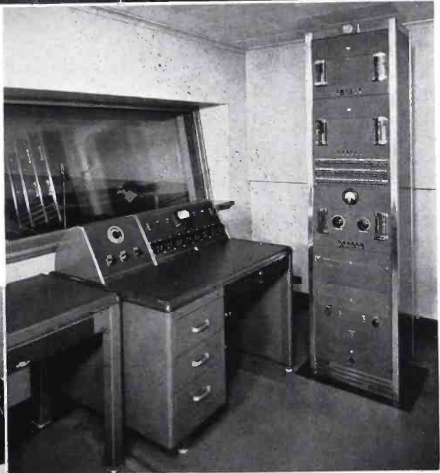
(Above) A Studio Control Console and Rack built for WFBR.
