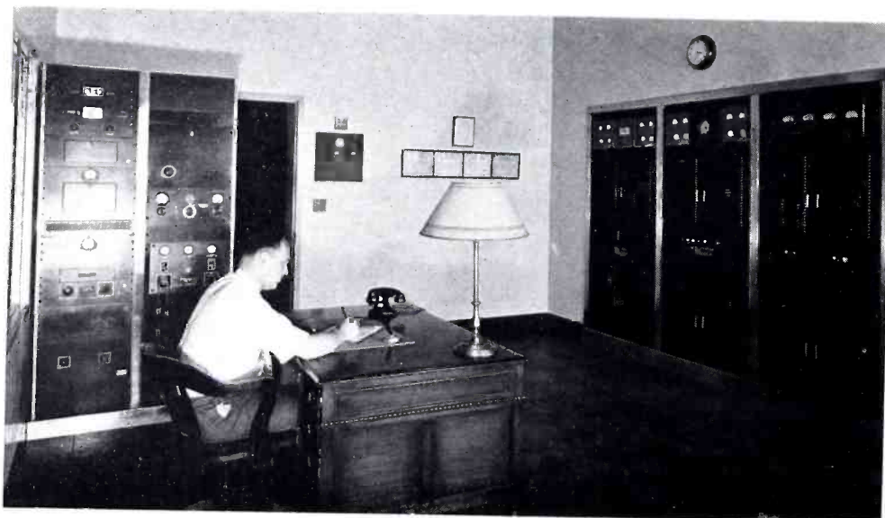
Below: WGR Operating Room with the RCA 5KW transmitter on the right.
