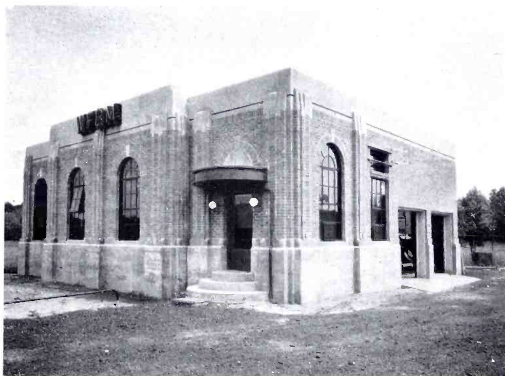
The compact and efficient plant which houses the transmitter.
