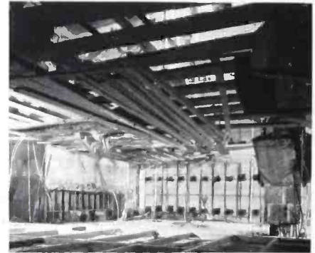
Figure 2. Reconstruction work in one of the old CBS studios.
