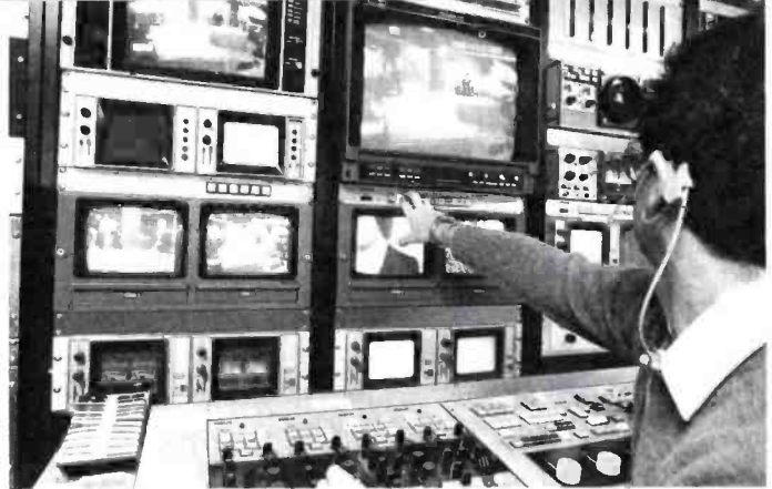
Set-up and remote controls for TK-47 cameras are located in Master Control.
