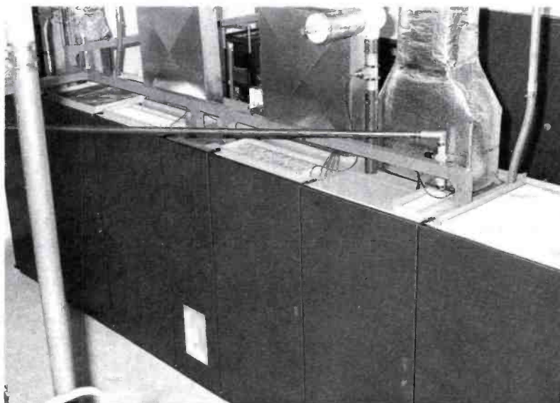
Optimized RF output switching unit—"OptoSwitcher"—provides for motorized switching of aural and visual transmitter outputs. Switches are packaged to allow for complete accessibility.
