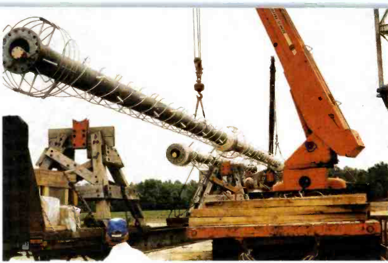
WBTW-TV's Tetracoil CP antenna was trucked from Gibbsboro, N.J. to the tower site at Dillon, S.C. in two pieces and was assembled on the ground.
