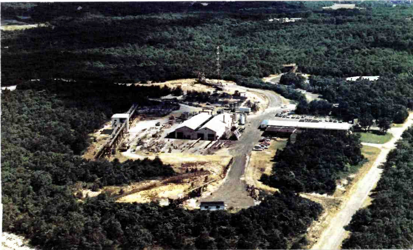
Aerial view of the RCA Antenna Engineering, Assembly and Test facility at Gibbsboro, N. J.
