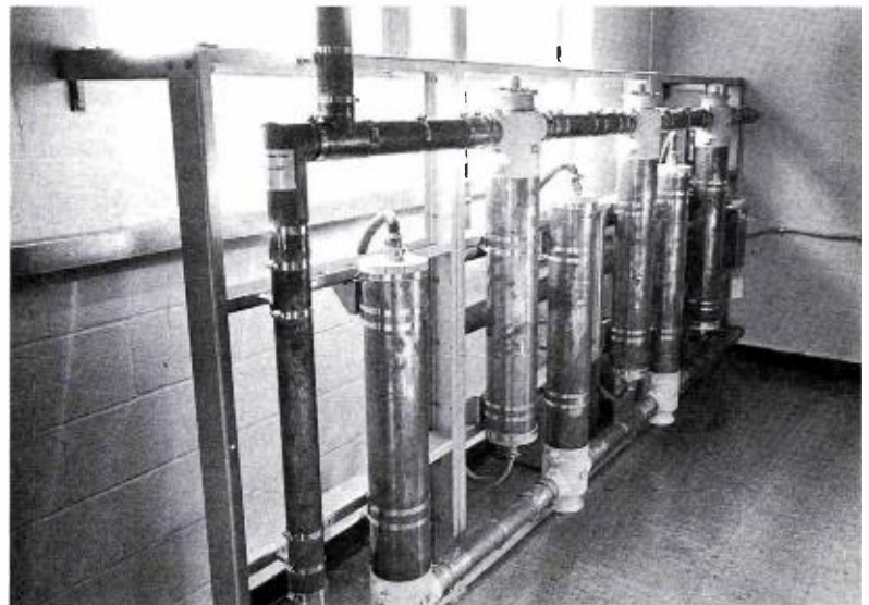
Wall-mounted Vistigial Sideband Filter for TT-50FL.
