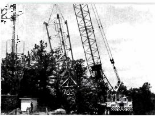
Crane hoists first section of 2,000 ft. WRAL tower into position.
