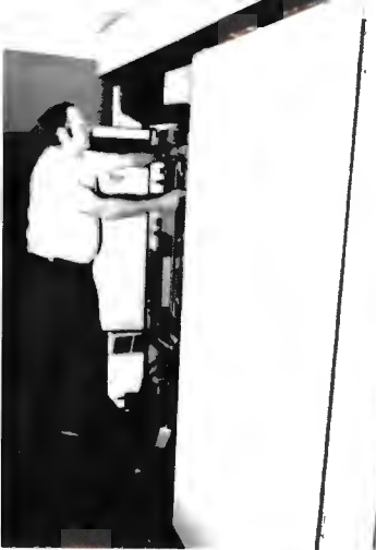
Maintenance Supervisor Ray Reome checks TCR-100. To fully utilize available space, the rear of the tape machines are serviced from the outside hallway. Sliding pegboard panels permit easy access.
