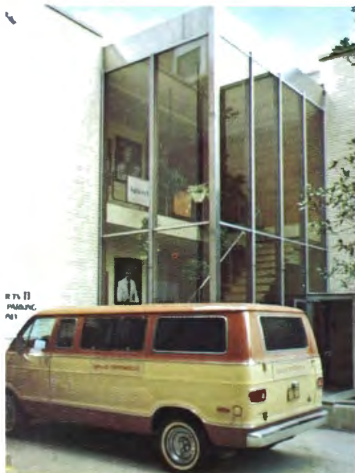
Glassed-in rear entrance for TV-11 News operation. In upgrading, KPLR-TV opted to stay at their in-town apartment location by revamping the technical operations and modernizing the total facility.
