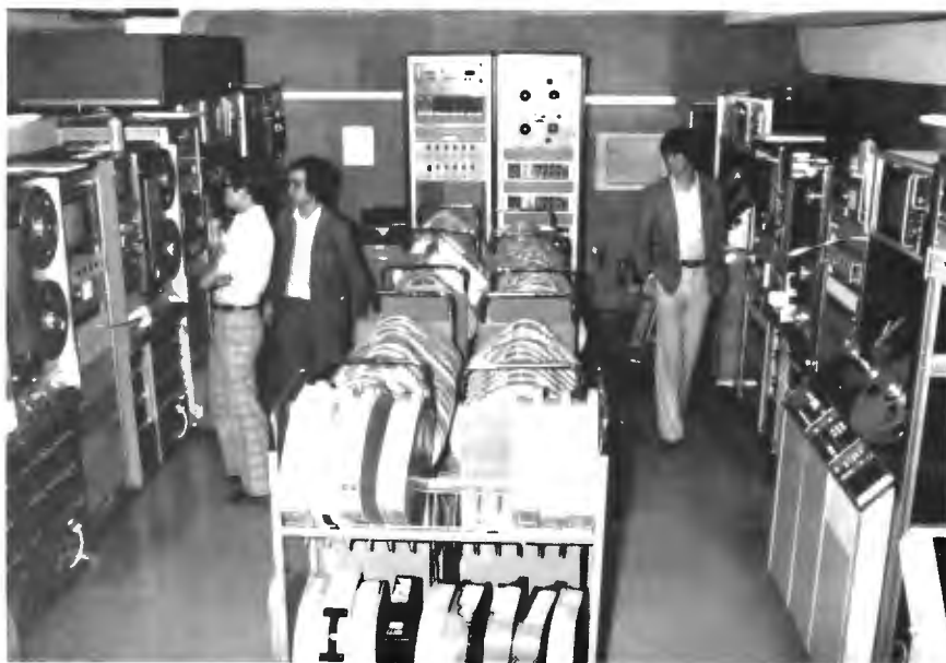
The VTR room has kept pace with RCA's developing tape line. Three TR-600's were recently added to meet the growing demand for local tape production.
