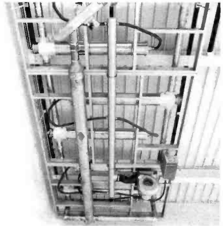
Ceiling-mounted 50 kW vestigial sideband filter.
