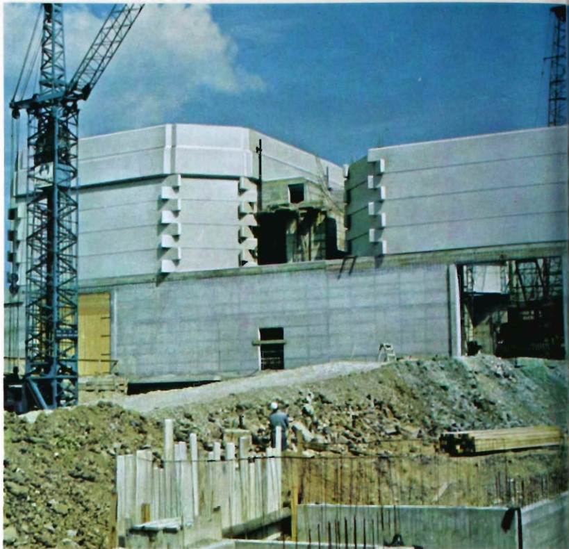
Fig. 12 Studios 2 and 3 during construction. The upper parts of the studio walls are reinforced-concrete sections assembled in log-cabin fashion.
