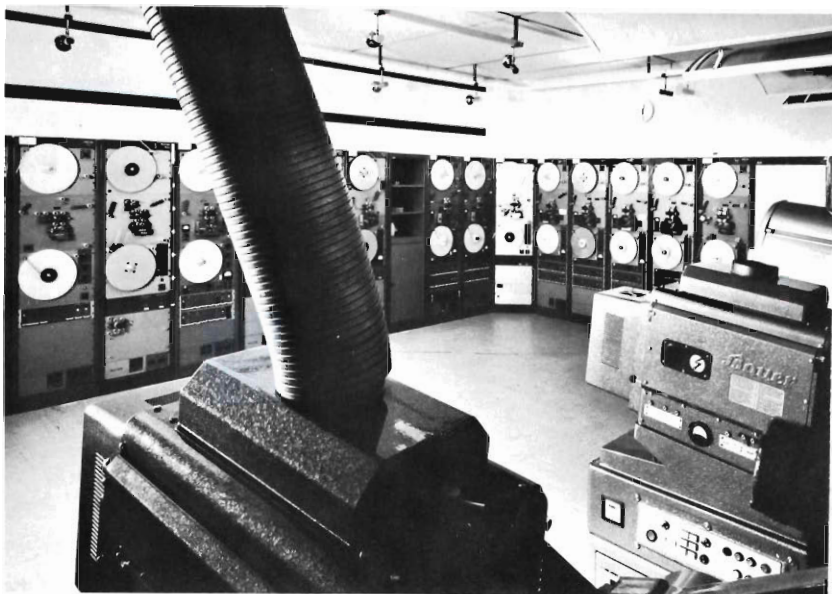
Fig. 28 One of the projection rooms in ORF's extensive sound dubbing facility. Film projectors which project film on to screen in dubbing studio are in foreground. At the rear are sound recorders used in dubbing and editing operations.
