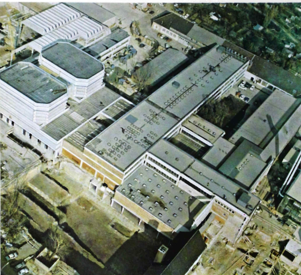
Fig. 19 In this view of the complex under construction, the low building (bottom, center) with the many skylights is the central machine room. The central equipment room and master control area is between the machine room and the studios. The area at the bottom left of this photo is where the main office building will go. From the first floor lobby of the office building the central machine room will be visible thru a larger glass wall.
