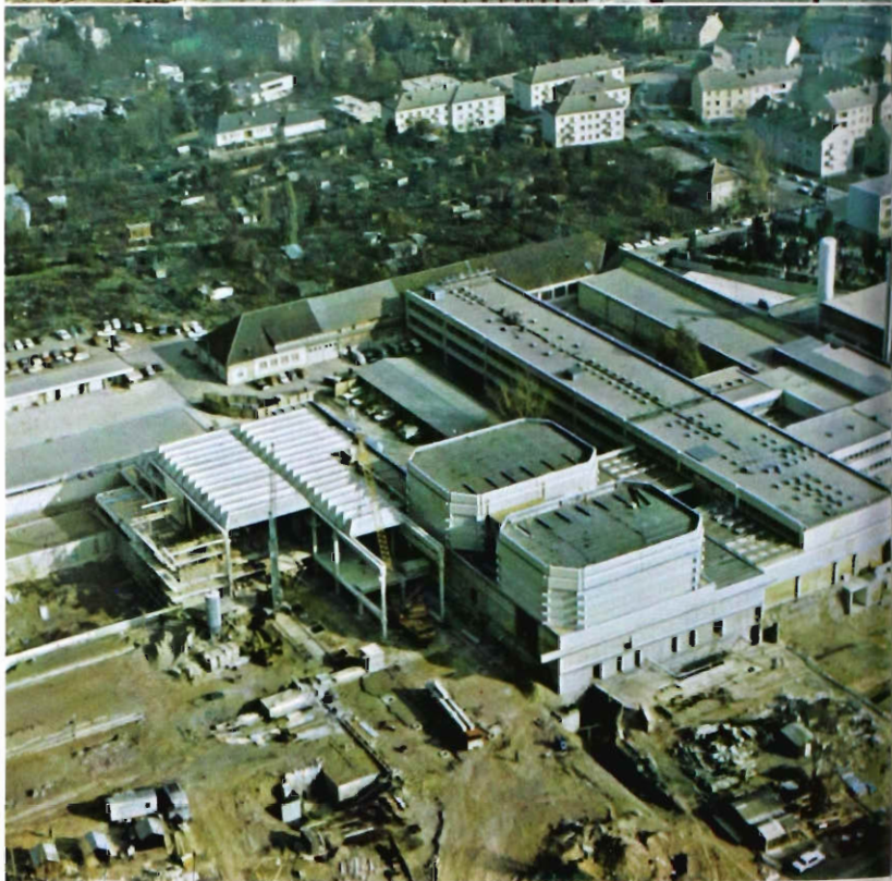
Fig. 13 Aerial view of construction progress. At this stage the scenery shops (lower, left) were partially completed. When finished they will extend out to abut the side of the TV theatre which will be in the area at the bottom center of this picture.
