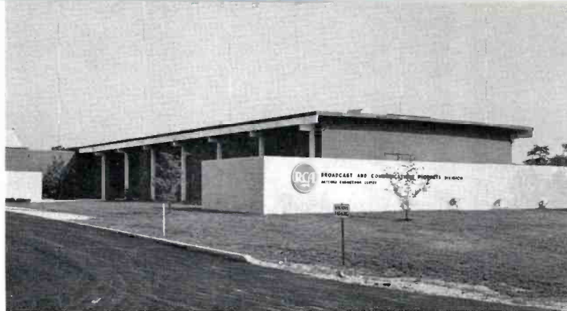
FIG. 8. Exterior view of the lab/office building. Note the wooden pillars which support laminated-wood girders which, in turn, support the all-wood roof. All wood construction assures accuracy of antenna tests.
