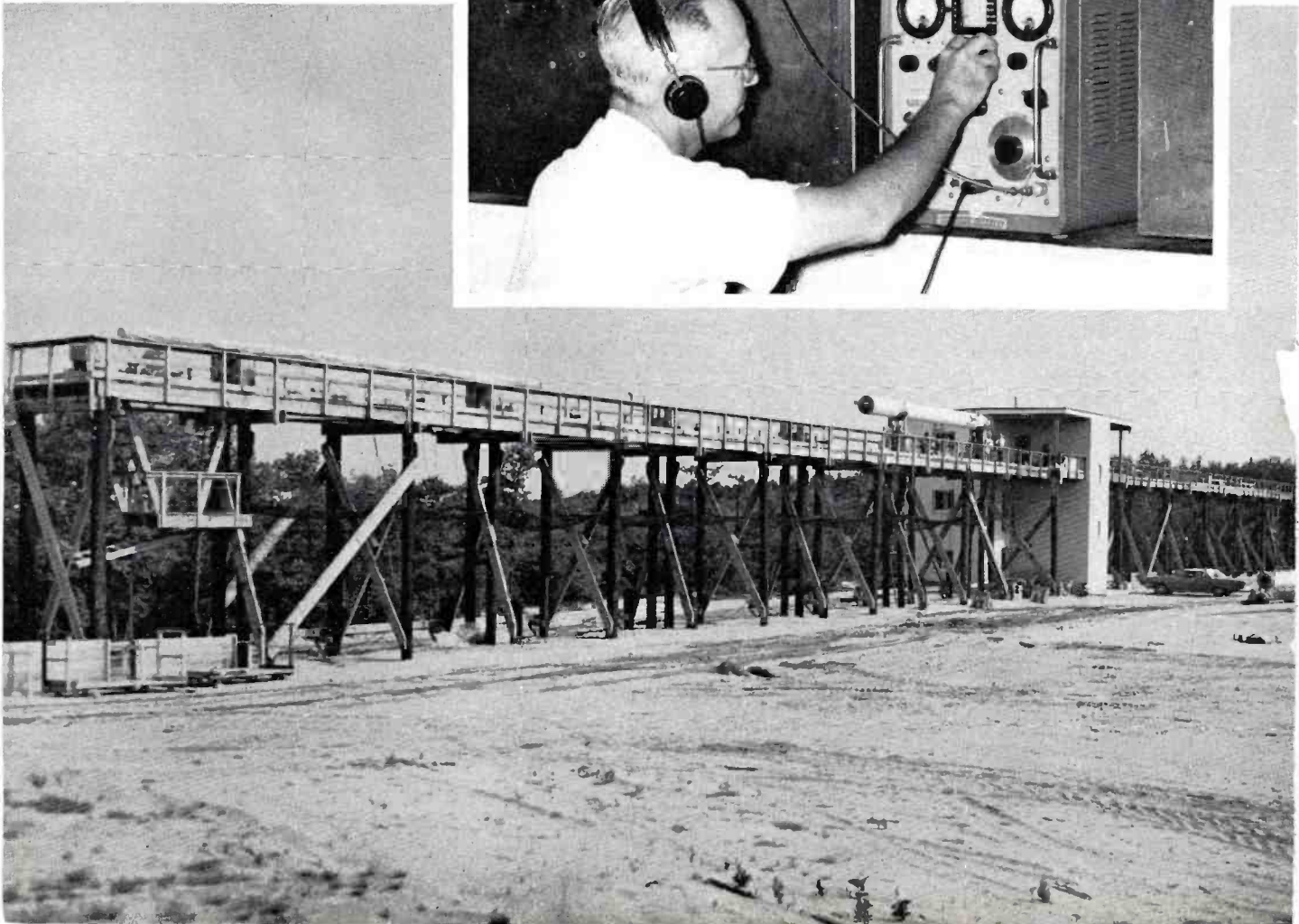
FIG. 14. The VHF antenna trestle measures almost 400 feet end-to-end. This structure is used in the test and final adjustment of traveling-wave and other VHF antennas. Test gear is in building at center. ▼
