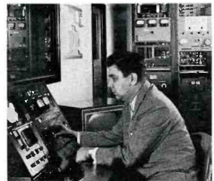
FIG. 26. Transmitter supervisor Bob Larson at transmitter control point, which also handles selection of diplexed microwave receivers.
