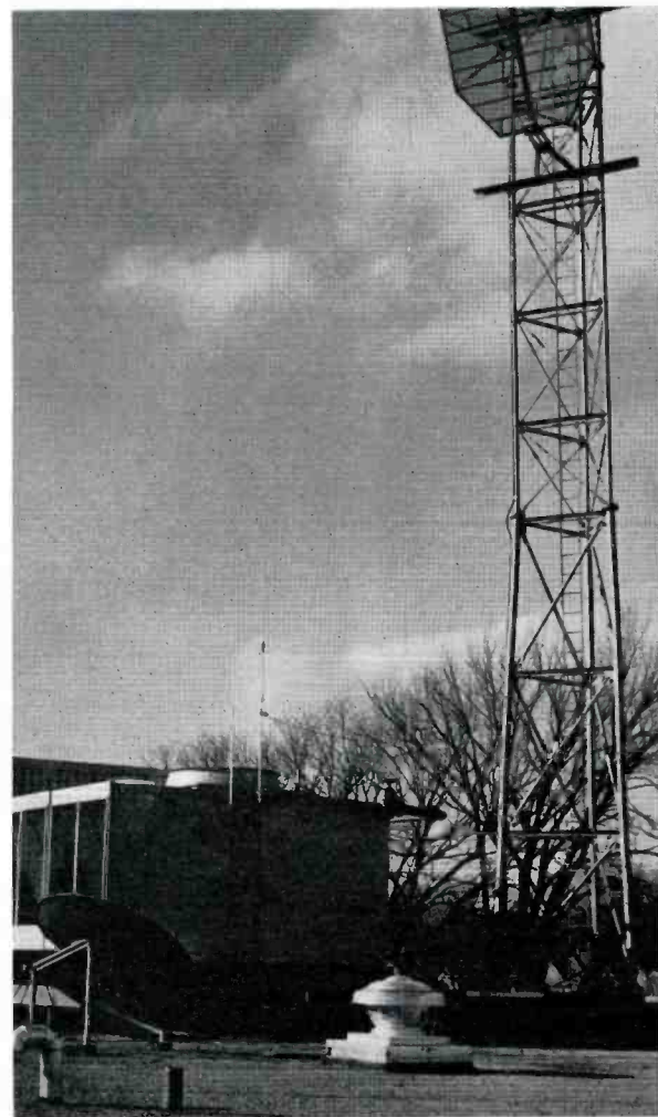
FIG. 25. On top of building is a 75-foot tower, mounting reflectors for the microwave relays of the telephone company which bring network and other outside programs into WQAD-TV master control and the STL over which programs are transmitted from the studio to the transmitter.
