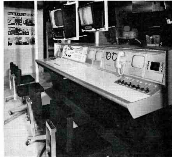
Functional new console . . . beginning of control room revolution.
