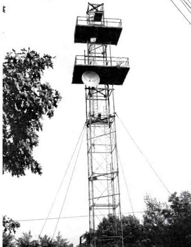
FIG. 8. This transmitting tower at Union Mills, located 2.4 miles from the turntables, emits the test signals.
