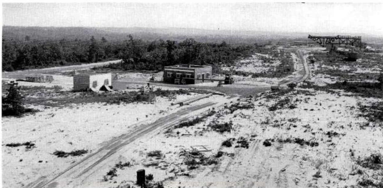
FIG. 5. The 15-ton antenna turntable is shown in the background of this over-all view of the RCA Antenna Testsite.
