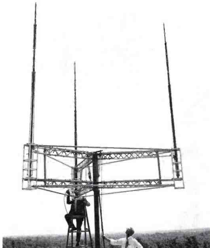
FIG. 10. Scale model of a Multiple Antenna arrangement, employing three superturnstile, undergoing test.
