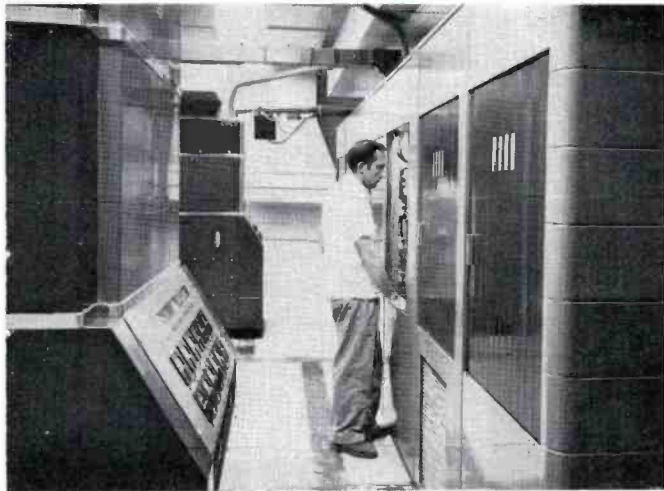
FIG. 29. Rear view of transmitter cubicles. At left, are 50-kw power amplifiers. Note generous aisle area.
