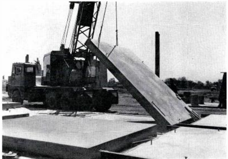
FIG. 5. Building is constructed of precast cement panels.
