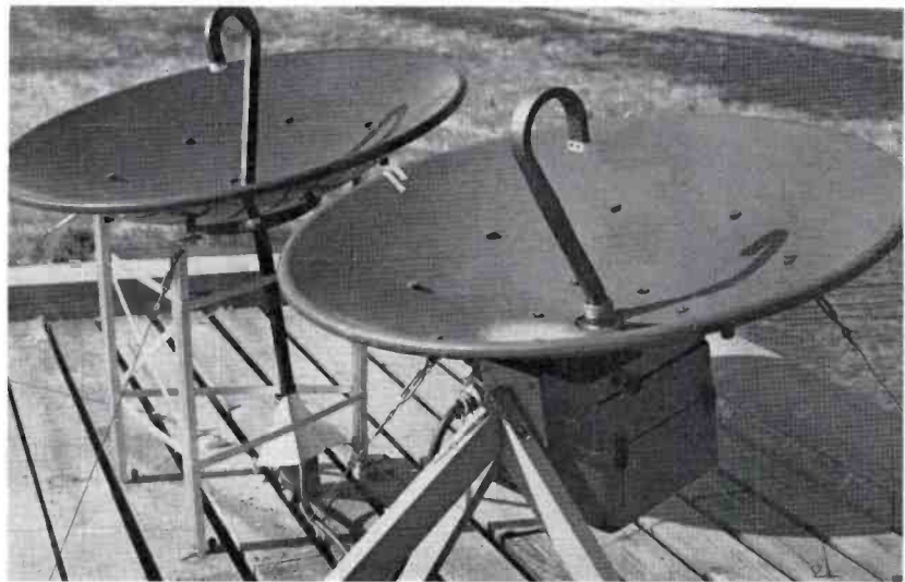
FIG. 24. (Left) STL link waveguide feeds directly through roof into video racks beneath. (Right) Remote pick-up microwave unit, placed on roof as STL standby when not in use for remote work.
