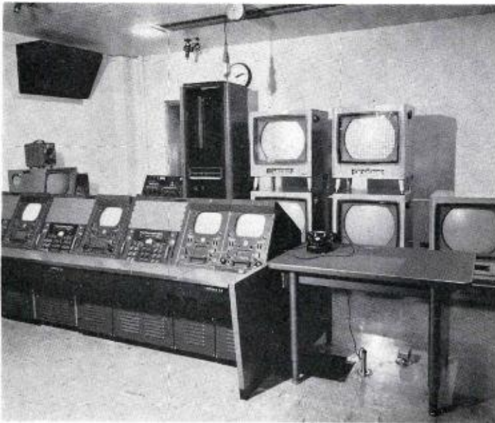
FIG. 7. View of front of control room showing camera controls and switching equipment, (left to right): (1 and 2) TK-26; (3 and 4) TK-45; (5 and 6) TK-41; and (7) TS-11 Switcher. Director's table is at right. Audio equipment is in left background and five color receivers used by directors are at right.
